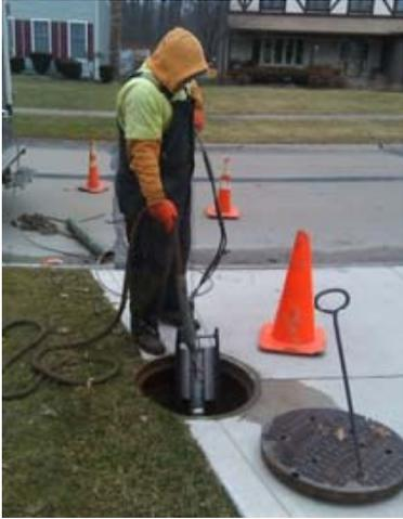
CCTV Utilized During Dye Testing
