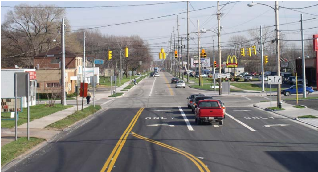
City of Lorain Colorado Avenue Improvements
