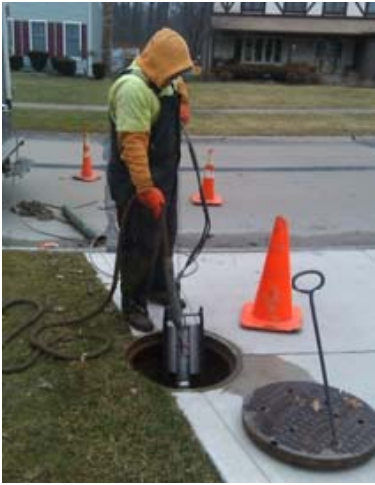
CCTV Utilized During Dye Testing
