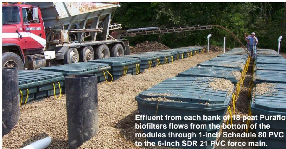
Effluent from each bank of 18 peat Puraflo biofilters flows from the bottom of the modules through 1-inch Schedule 80 PVC to the 6-inch SDR 21 PVC force main.
