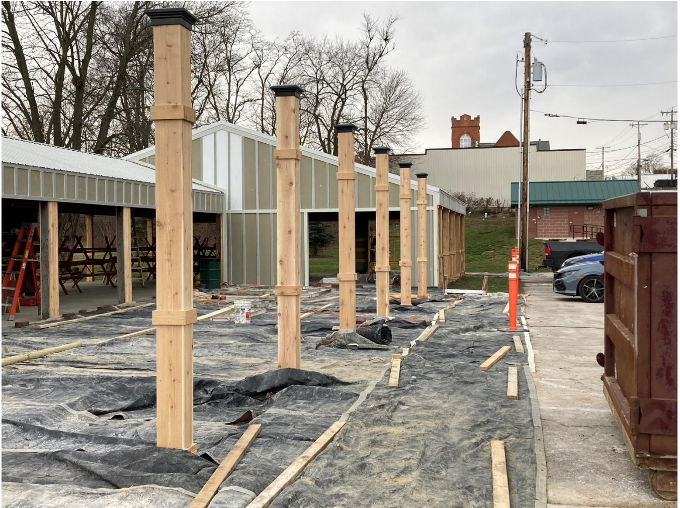
Covered concrete slab at shelter area w/new cedar wrapped posts in foreground
