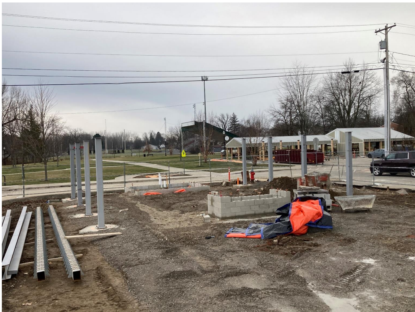
Structural steel at pergola w/foundations of fireplace and pumphouse visible
