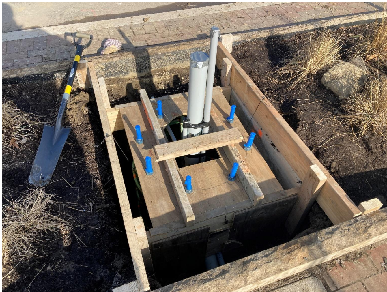
South arch foundation pre-pour facing north
