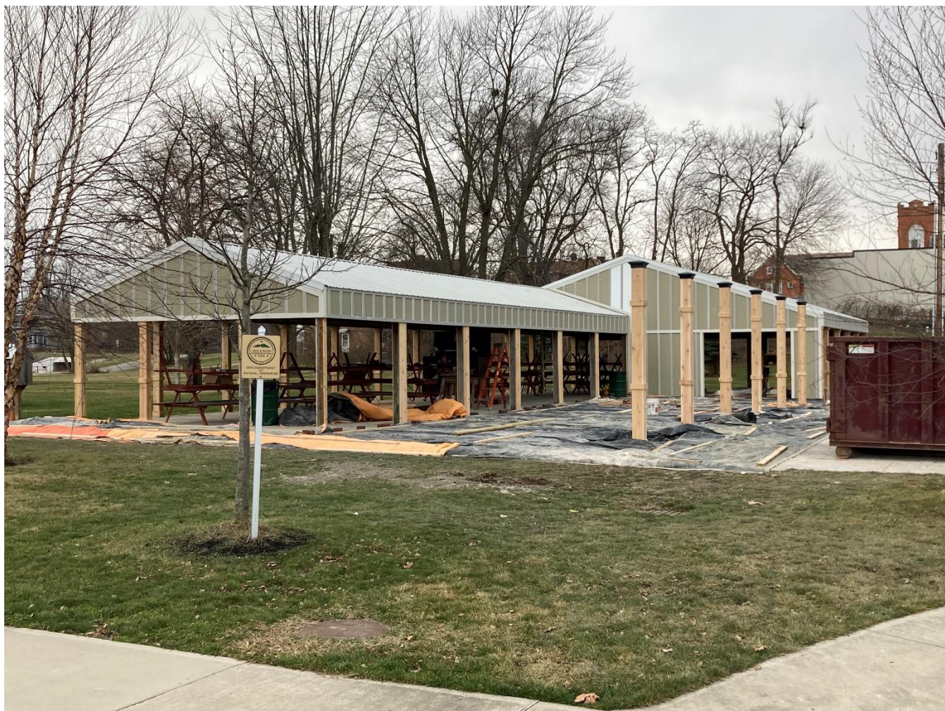
Existing pavilion w/new Hardie board and batten
