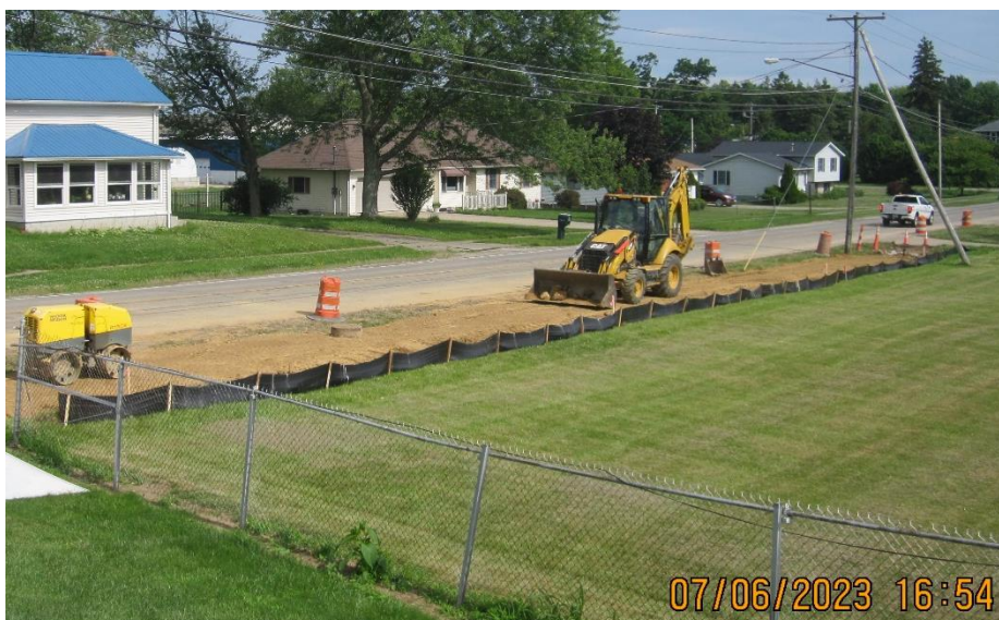
Thursday July 6 th : Compacted Subgrade of North Sidewalk Section.
