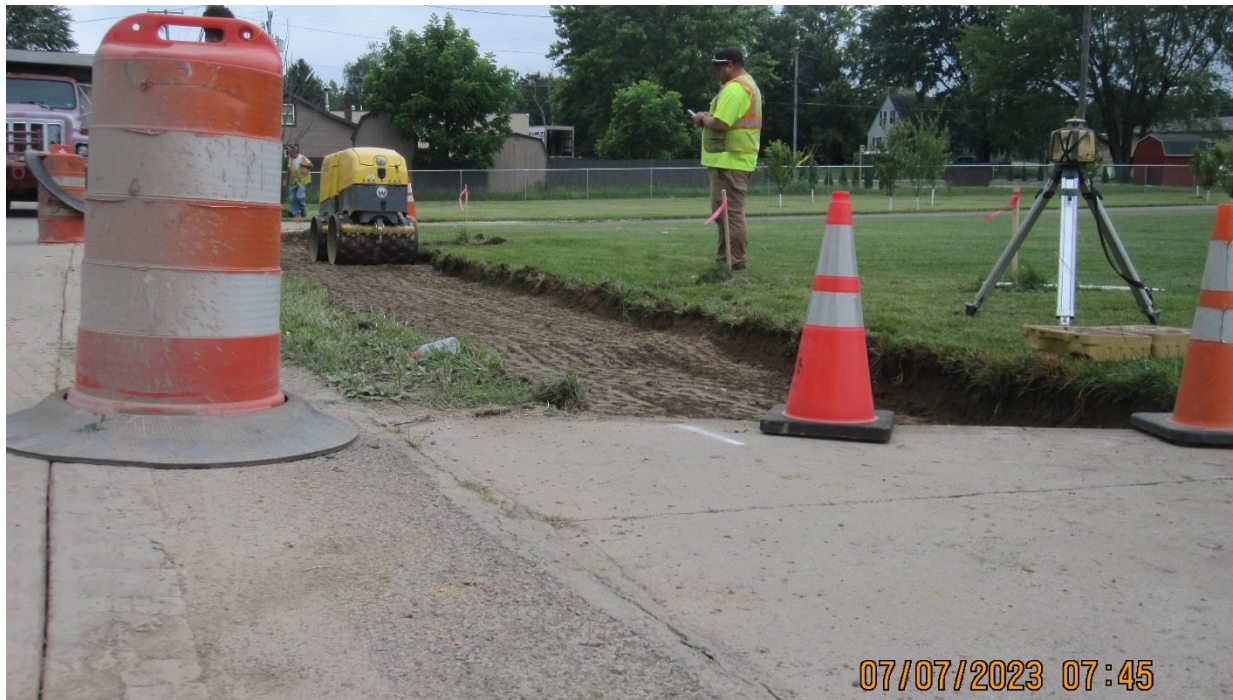
Friday July 7 th : Compacted Subgrade of South Sidewalk Section.
