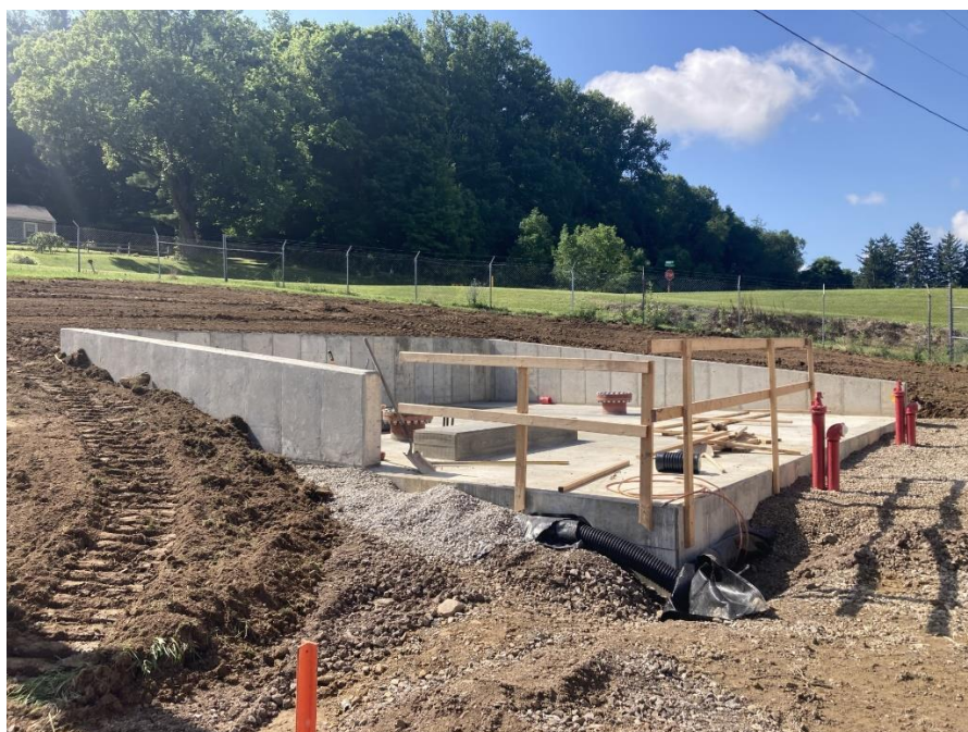
Grading at surge tank pad.
