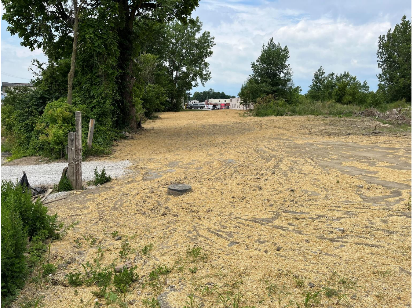
Straw placed after seeding.
