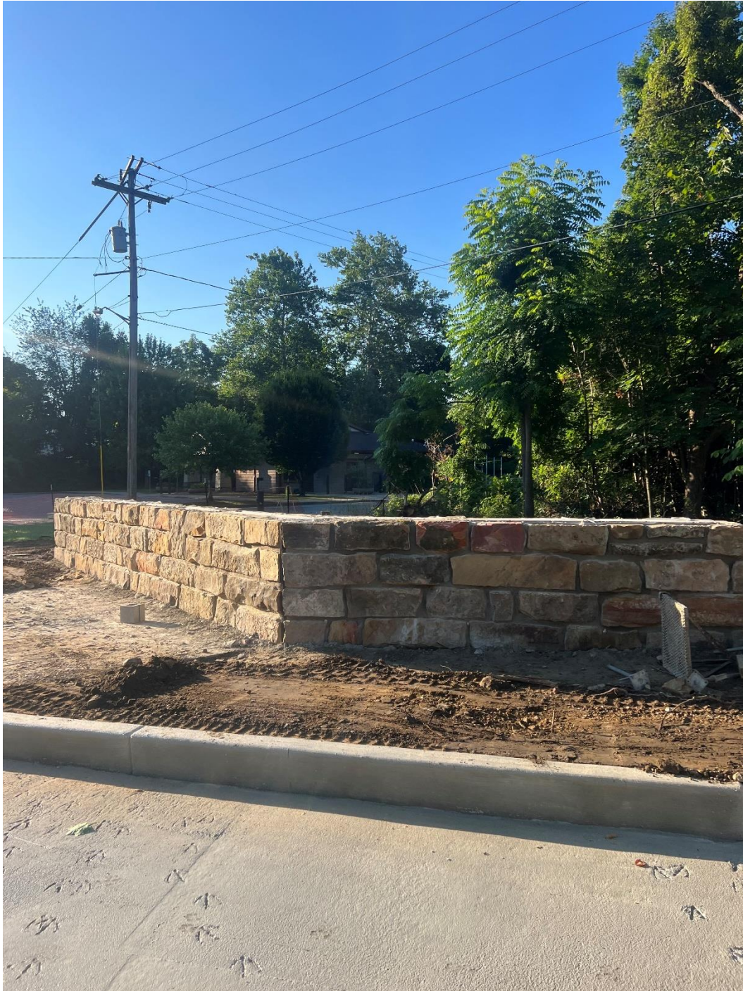
Sandstone on the inlet walls.
