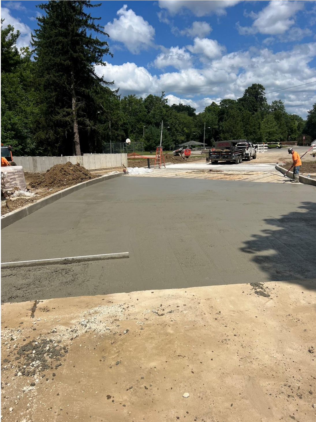
8" concrete base under roadway.
