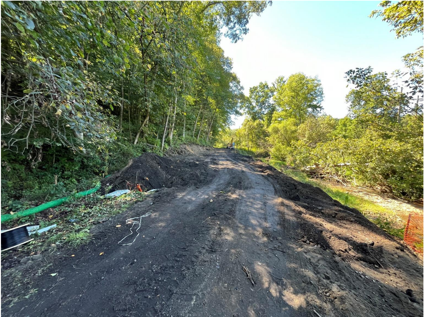
Wall 7 excavation/ staking.
