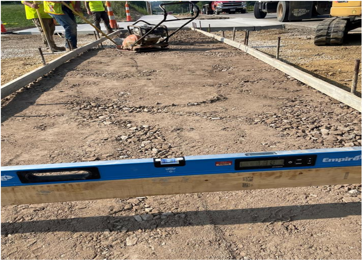
Wednesday August 28 th : SW-4 Cross Slope Check
