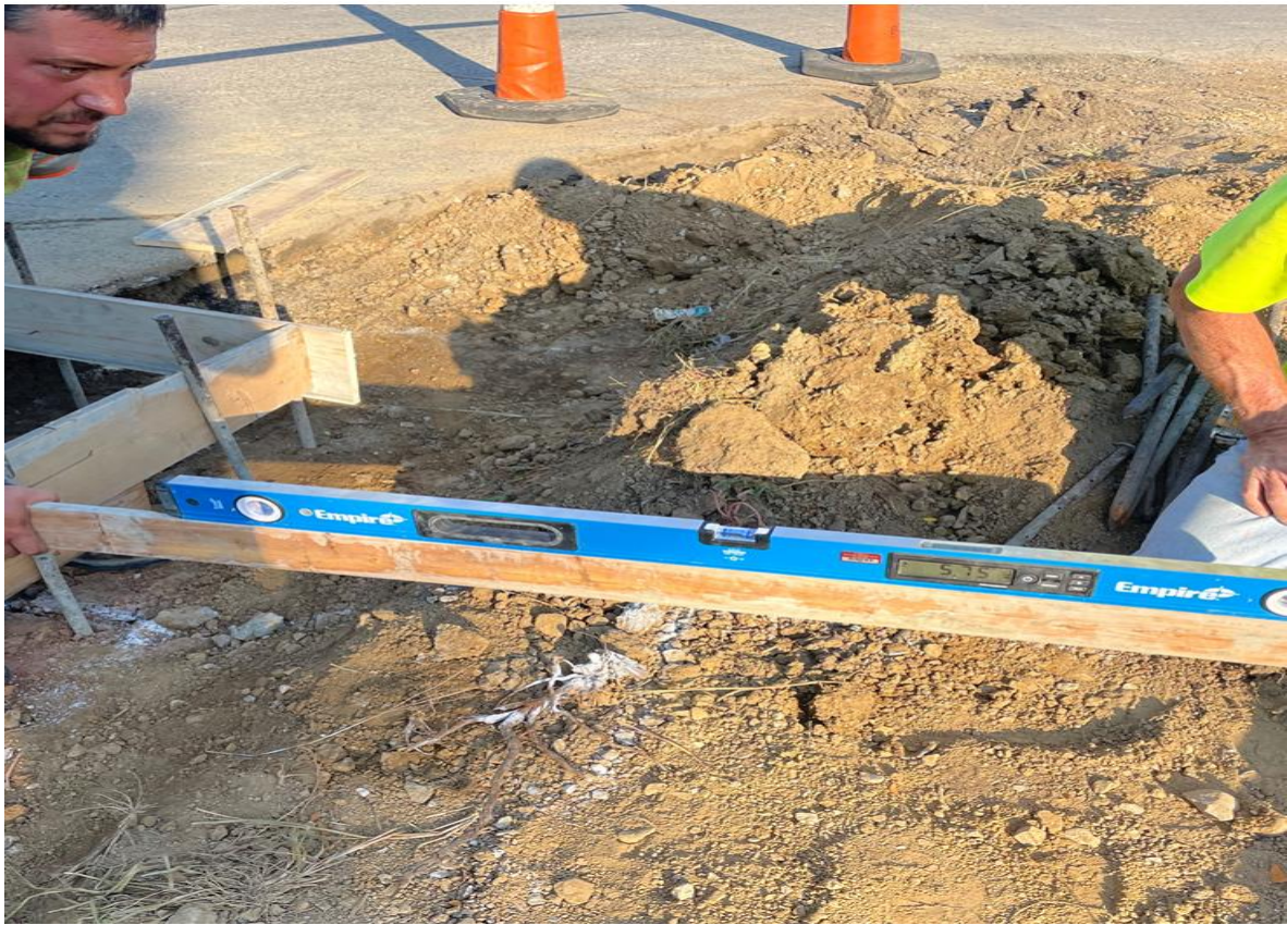
Friday August 30 th : CR-2 Ramp Running Slope Check
