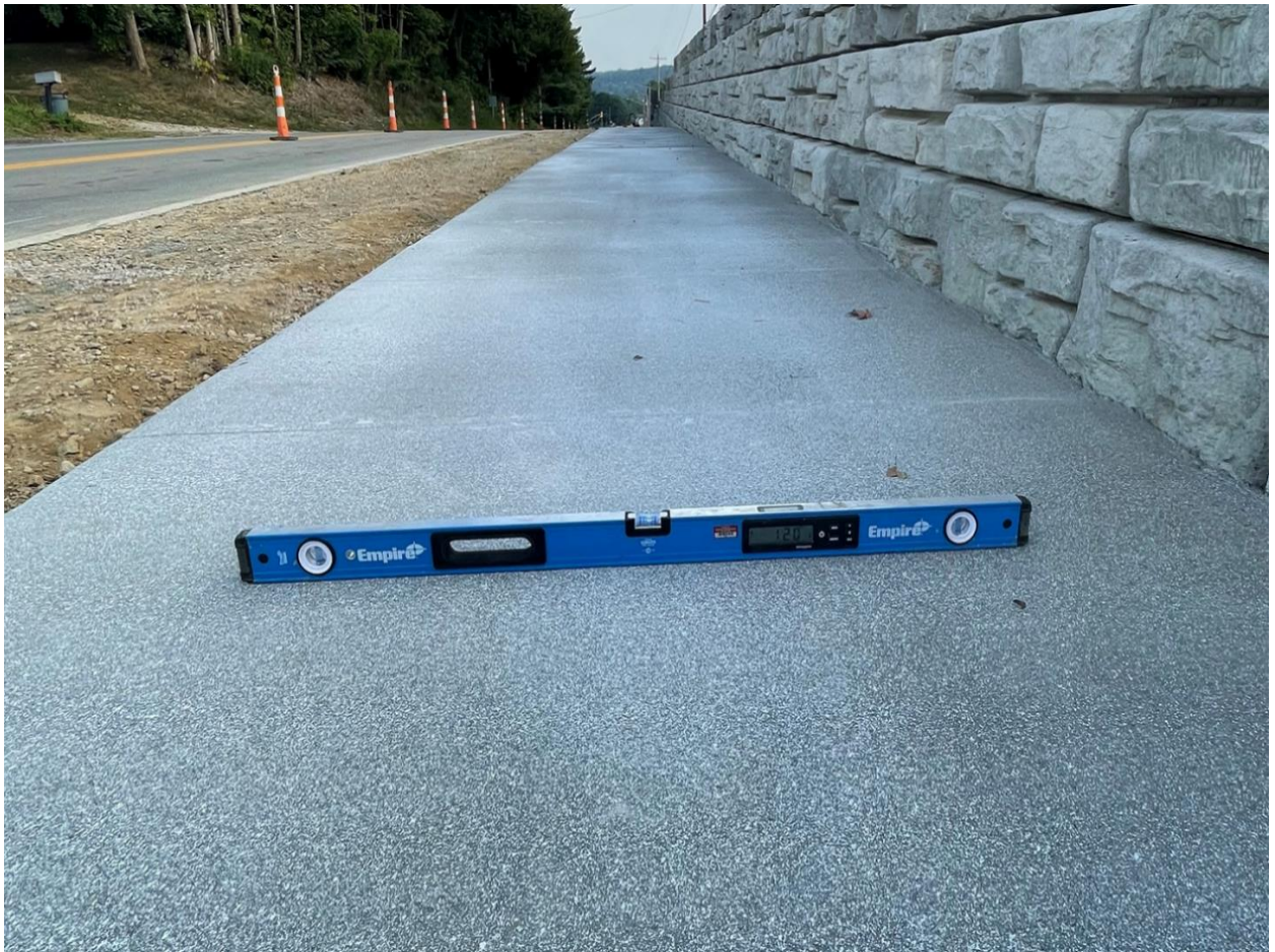
Monday August 26 th : SW-4 Wall Cross Slope Check
