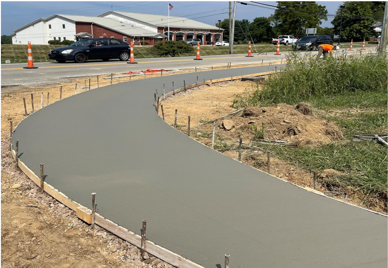
Tuesday August 27 th : SW-3 Poured
