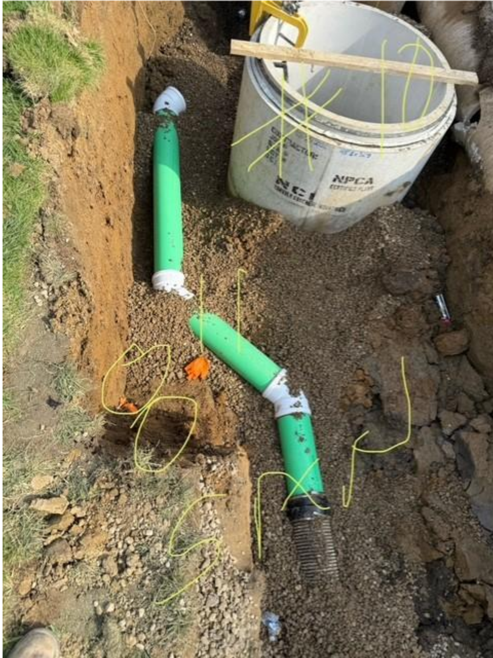
Existing Sanitary Replacement
